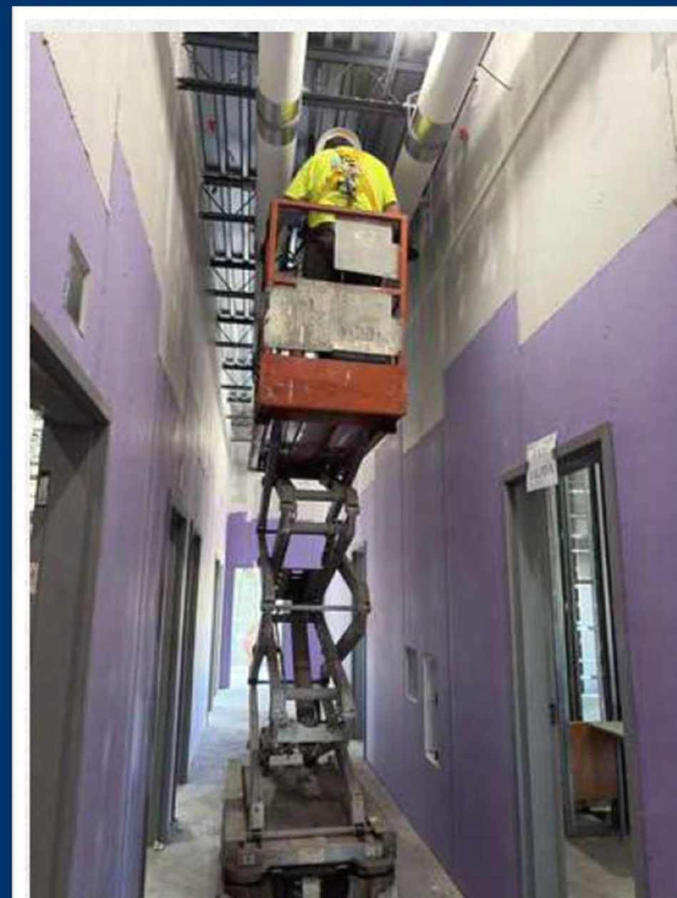
Taping and mudding of sheetrock in Corridor
